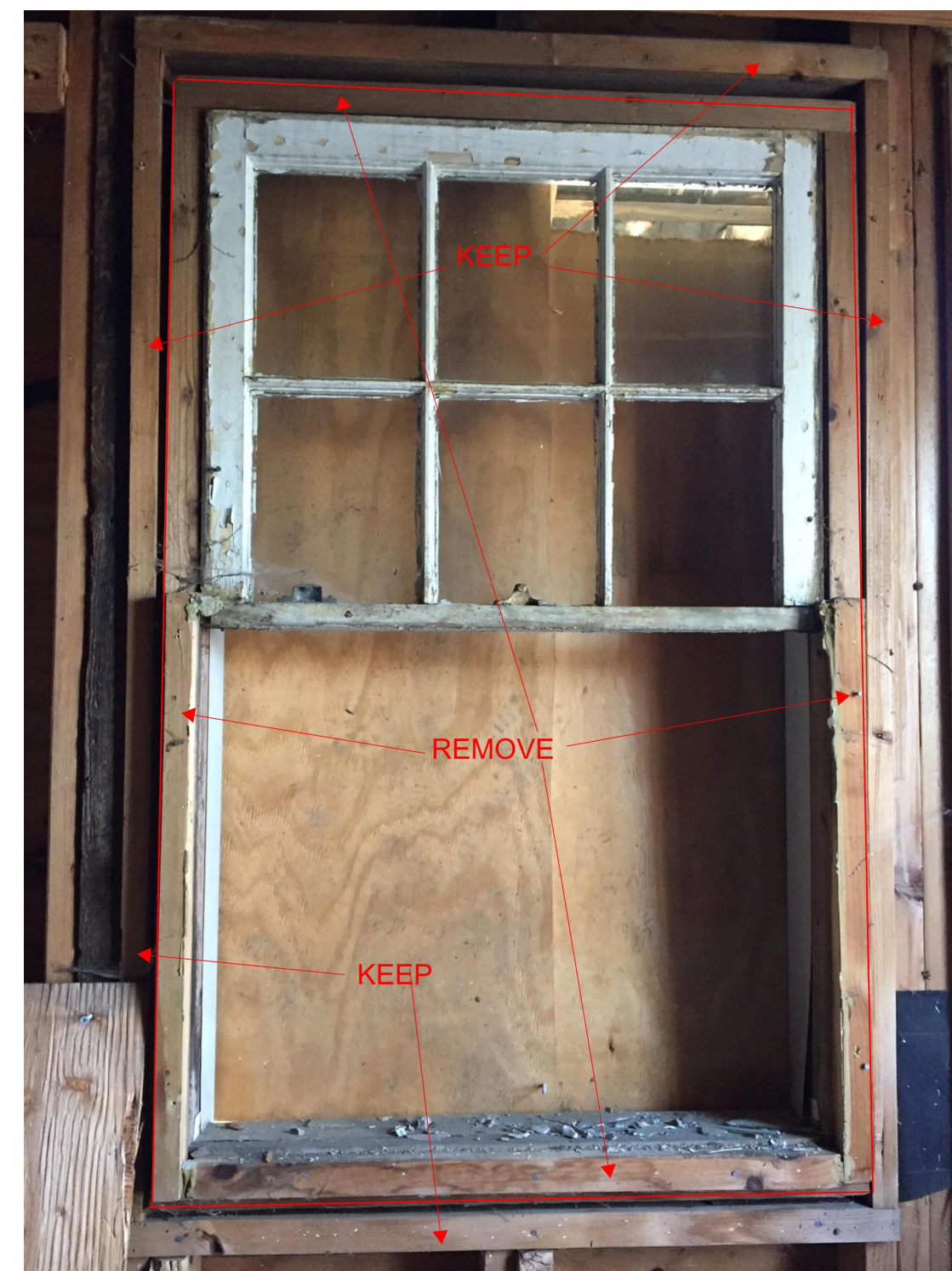
SEE ABOVE PHOTO AT EXISTING WINDOW. REMOVE EXISTING WOOD FRAME AS INDICATED.
