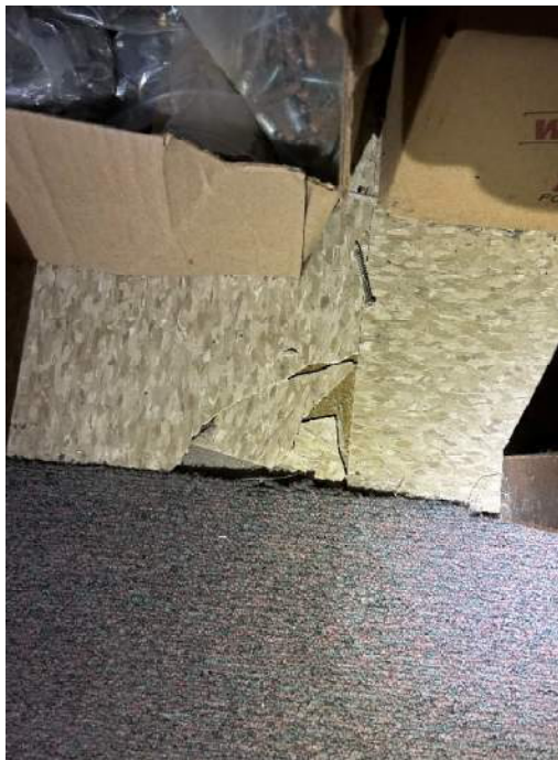
Photograph 19: HID 21. 12"x12" Gray Marbled Floor Tile (NAD) and Mastic (NAD)
