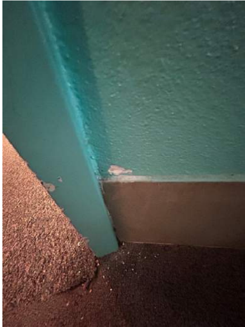
Photograph 17: HID 19. CMU Wall Parging (ACM)
