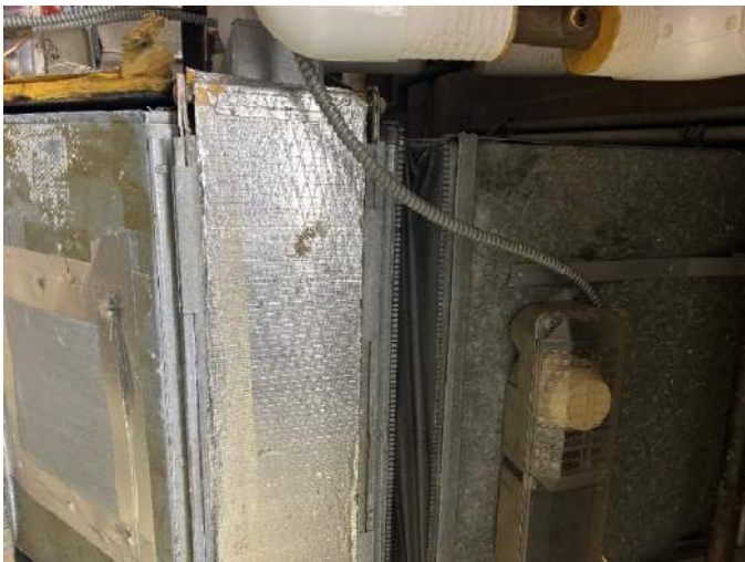
Photograph 7: HID 06. Black Vibration Dampener (Not Sampled/Assumed ACM)
