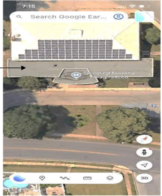
Photograph 22: HID 24. Roofing Material ( Not Sampled/Assumed ACM ), Front Roof
