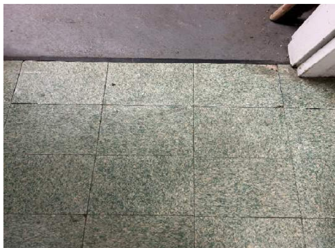
Photograph 2: HID 01. 9"x9" Green Marbled Floor Tile (ACM) and Mastic (NAD)
