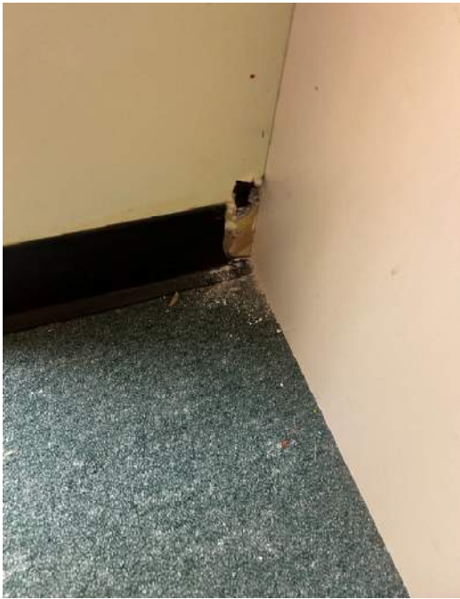
Photograph 9: HID 09. Black Covebase Molding (NAD) and Mastic (NAD) and HID 11. Drywall (NAD)
