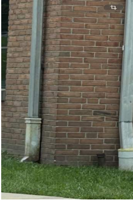
Photograph 21: HID 23. Exterior Brick Mortar (NAD)
