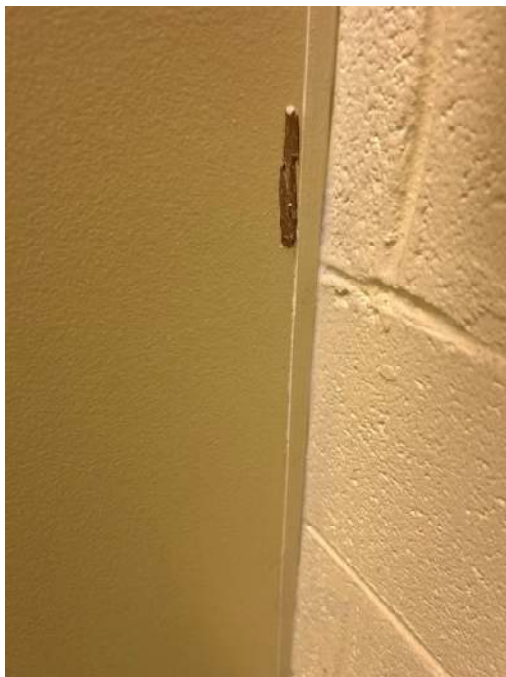
Photograph 11: HID 12. Joint Compound (NAD)
