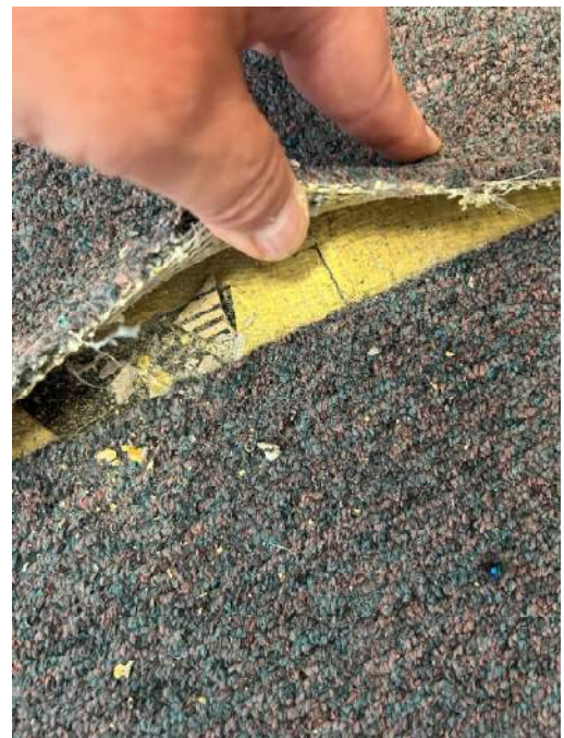
Photograph 8: HID 08. 9"x9" Beige Floor Tile (NAD) and Mastic (NAD)
