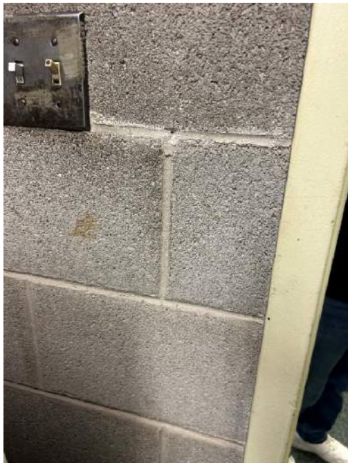
Photograph 15: HID 16. CMU Mortar (NAD)
