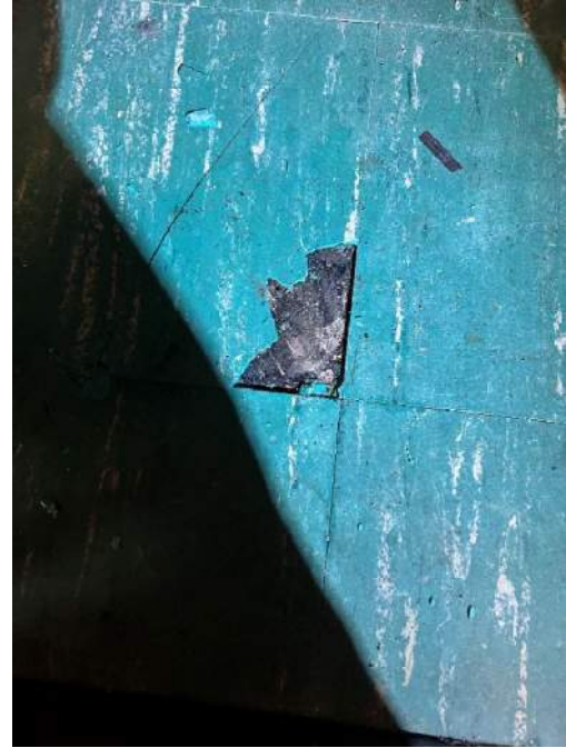
Photograph 18: HID 20. 9"x9" Green Streaked Floor Tile (ACM) and Mastic (NAD)
