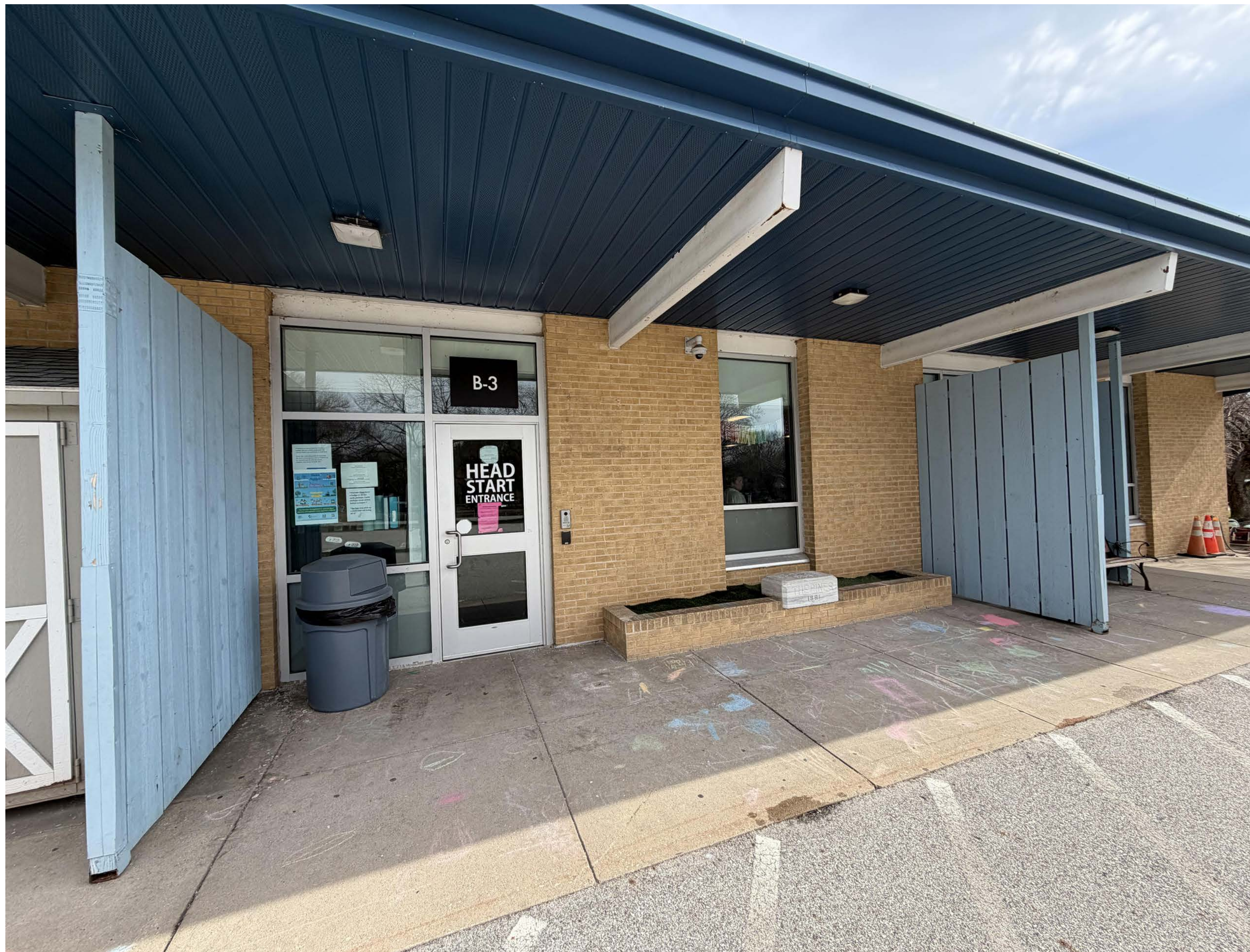
EXISTING BUILDING ENTRY
