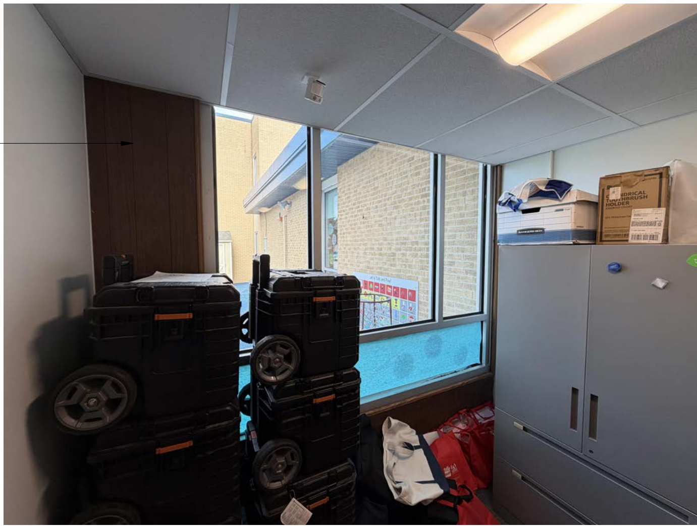
14 EXISTING OFFICE A-155 - WALL AREA NTS
