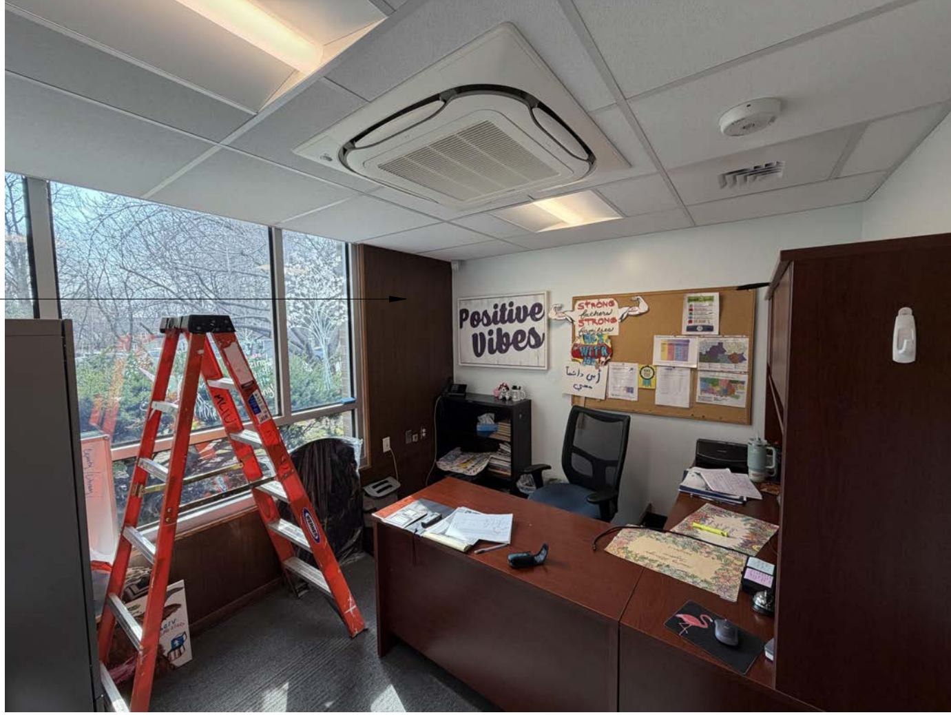
11 EXISTING OFFICE A-103 - WALL AREA NTS
