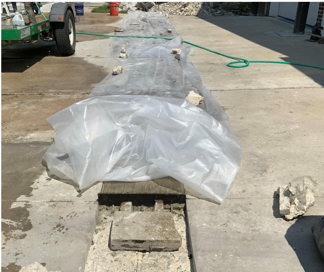
Photo 1: Summer 2023 Construction Progress of 2" Deep Topside Repair at Middle of Apron
