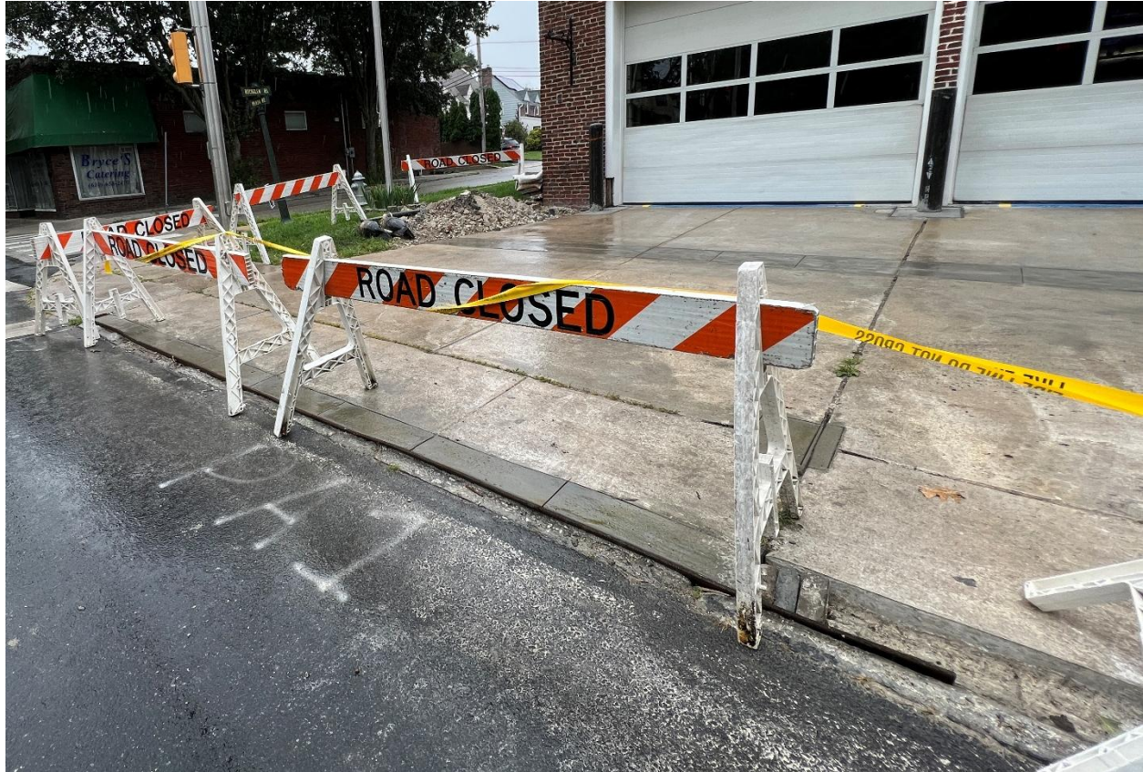
Photo 2: Summer 2023 Construction Progress of Topside Repair at Apron Edge
