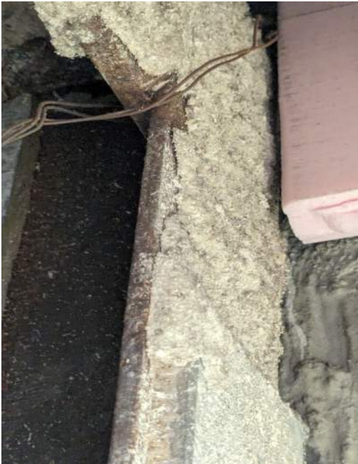
Photograph 20: HID 31. Spray Applied Fireproofing (NAD), 1 st Floor
