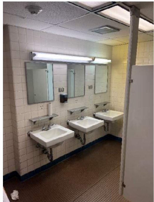
Photograph 40: HID 28. Mirror Adhesive (Not Sampled/Presumed ACM)
