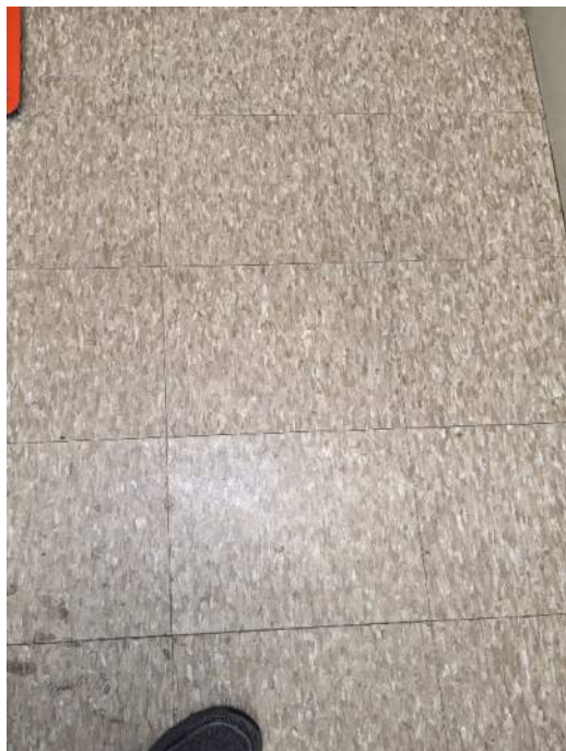
Photograph 25: HID 36. 12"x12" Brown with Tan Flake Floor Tile (NAD) and Mastic (ACM)
