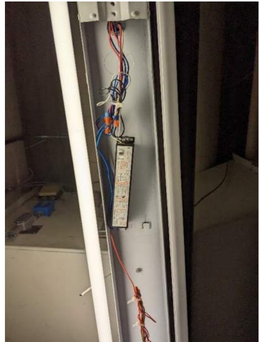
Photograph 48: Non-PCB Ballast
