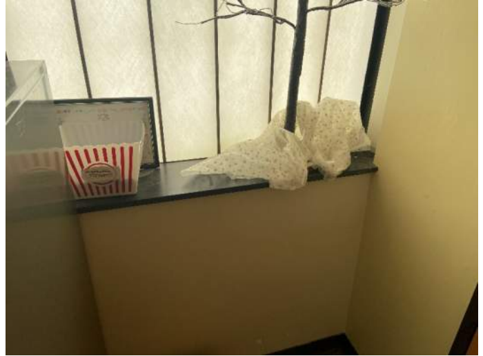
Photograph 14: HID 23. Black Cement Window Sill (ACM)
