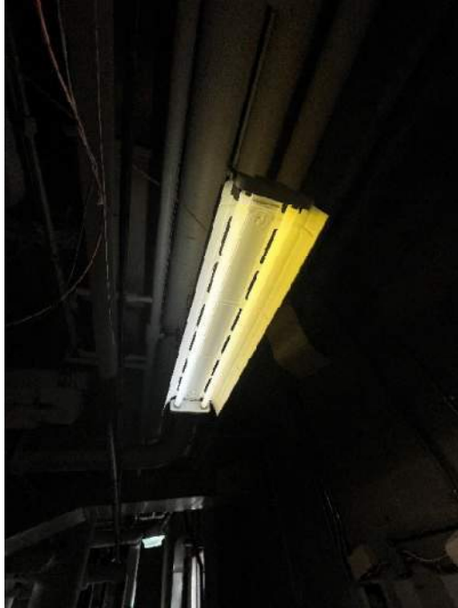
Photograph 45: 4-Foot PCB Ballast
