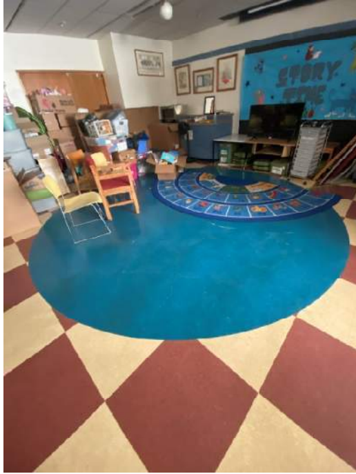
Photograph 17: HID 24. 12"x12" Tan Floor Tile (NAD) and Mastic (NAD); HID 25. 12"x12" Maroon Floor Tile (NAD) and Mastic (NAD); and HID 27. 12"x12" Blue Floor Tile (NAD) and Mastic (NAD)
