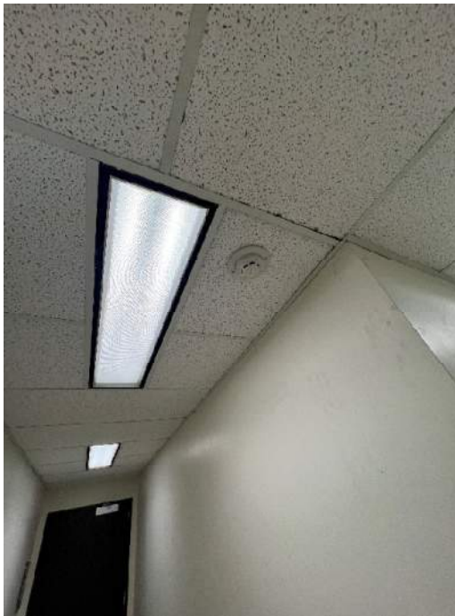
Photograph 51: Smoke Detector
