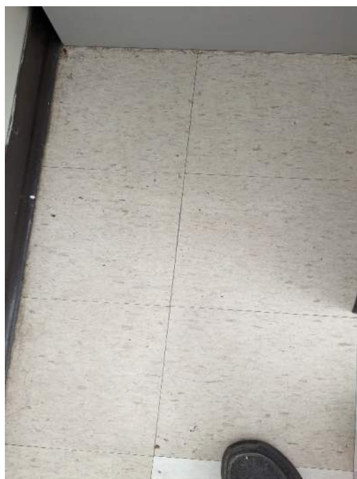
Photograph 12: HID 14. 12"x12" Tan and Gray Marble Floor Tile (ACM) and Mastic (ACM)
