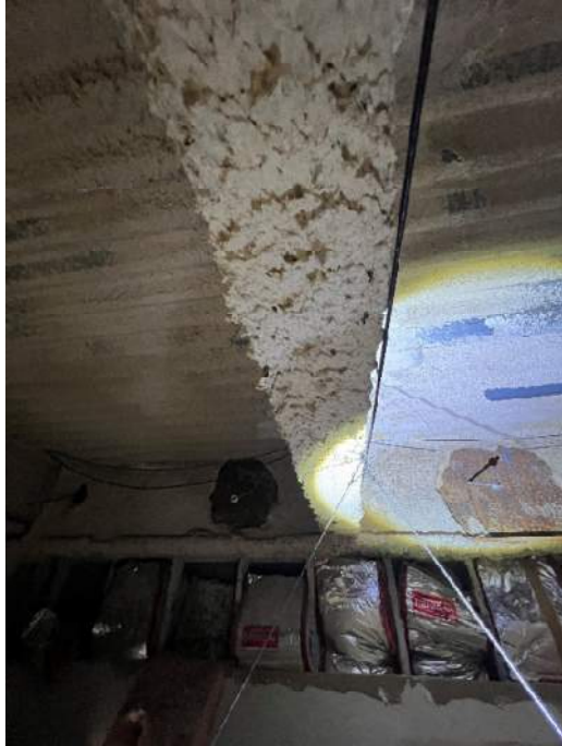
Photograph 33: HID 08. Off-White Spray-Applied Fireproofing (NAD) View above drop ceiling.
