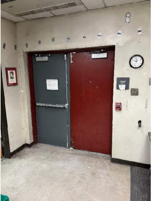
Photograph 34: HID 13. Fire Doors (Not Sampled/Presumed ACM)
