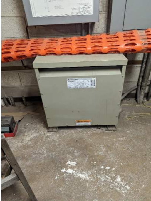
Photograph 57: Dry Transformer
