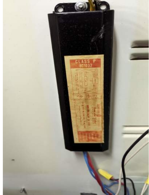
Photograph 46: PCB-Ballast
