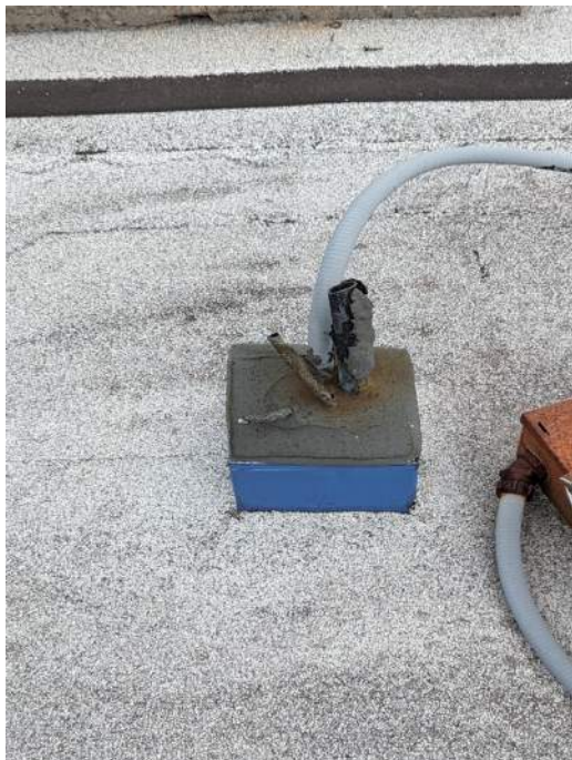
Photograph 43: HID 44. Roof Pitch Pocket (Not Sampled/Presumed ACM)
