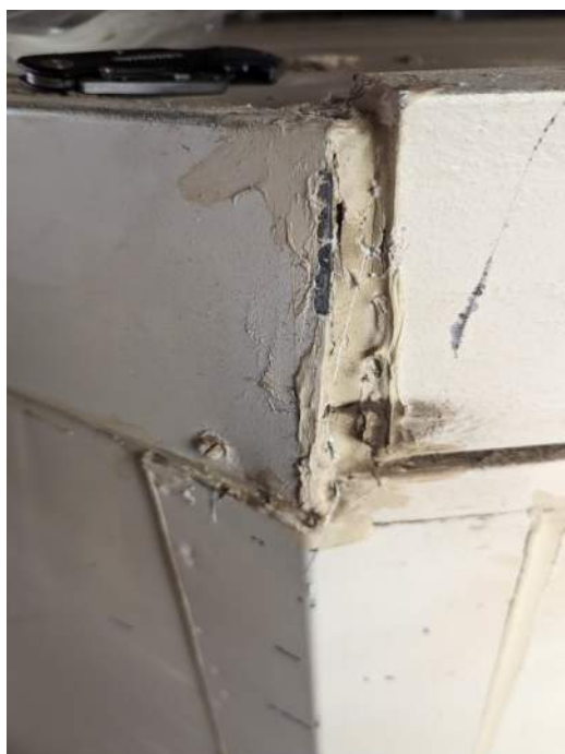
Photograph 11: HID 11. Joint Compound (NAD) and HID 12. Drywall (NAD)
