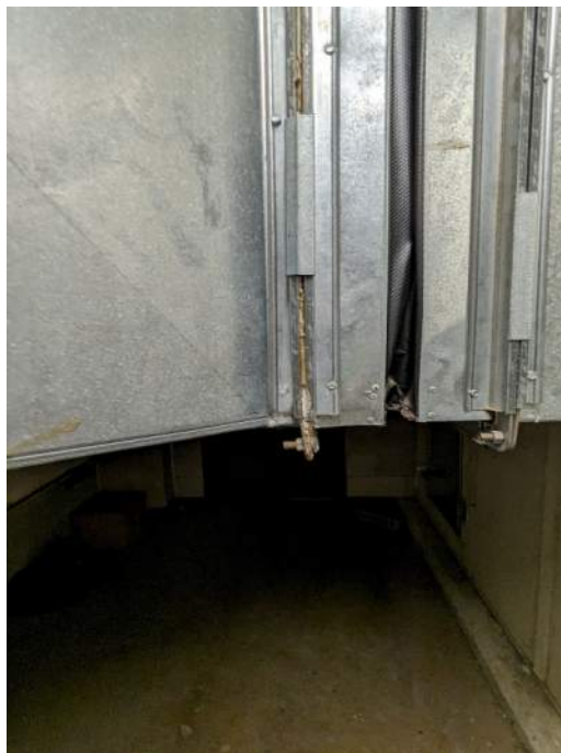
Photograph 65: Non-suspect asbestos-containing material
