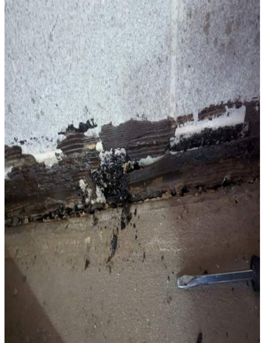
Photograph 6: HID 05. Dark Brown Covebase Mastic (NAD)
