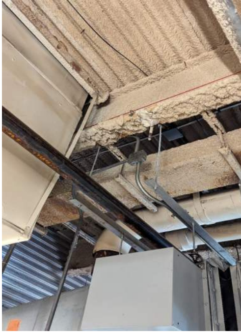
Photograph 1: HID 01. Tan Spray-Applied Fireproofing (NAD)
