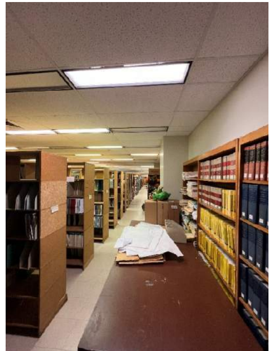
Photograph 16: HID 14. 12"x12" Tan and Gray Marble Floor Tile (ACM) and Mastic (ACM), Pictured in 2 nd Floor, Closed Stack Room
