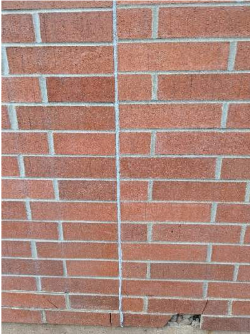
Photograph 29: HID 40. Exterior Brick Expansion Caulk (NAD)
