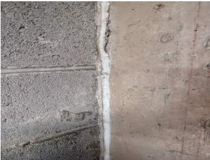
Photograph 4: HID 03. Expansion Caulk (NAD)
