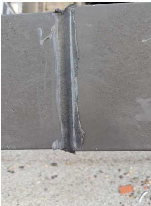
Photograph 28: HID 39. Capstone Metal Cap Caulk (NAD)
