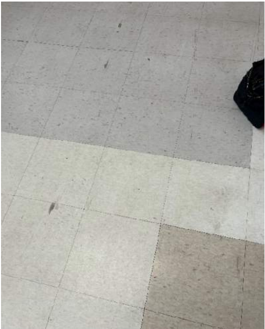
Photograph 36: HID 14. 12"x12" Tan and Gray Marble Floor Tile (ACM) and Mastic (ACM); HID 15. 12"x12" White and Gray Marble Floor Tile (NAD) and Mastic (ACM); HID 16. 12"x12" Gray and Brown Marble Floor Tile (NAD) and Mastic (ACM)
