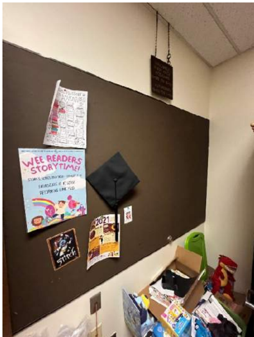
Photograph 39: HID 22. Wall Board Adhesive (Not Sampled/Presumed ACM)
