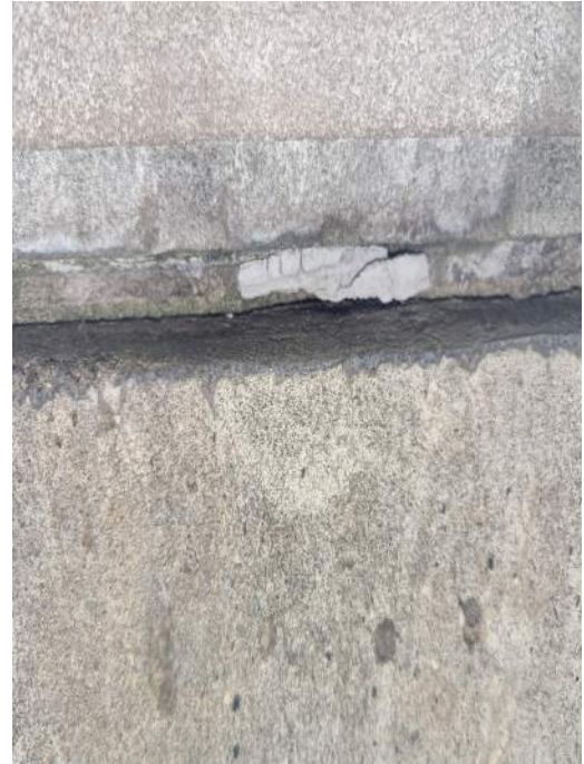
Photograph 30: HID 46. Exterior Concrete Wall Expansion Caulk (ACM)
