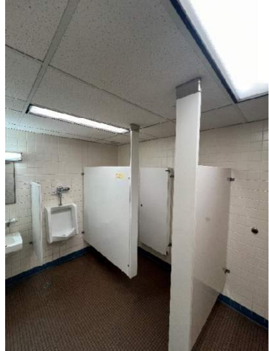
Photograph 38: HID 18. Ceramic Floor Wetbed (NAD); HID 19. Ceramic Wall Adhesive (NAD); and HID 20. 2'x4' Smooth Dot Ceiling Tile (NAD)
