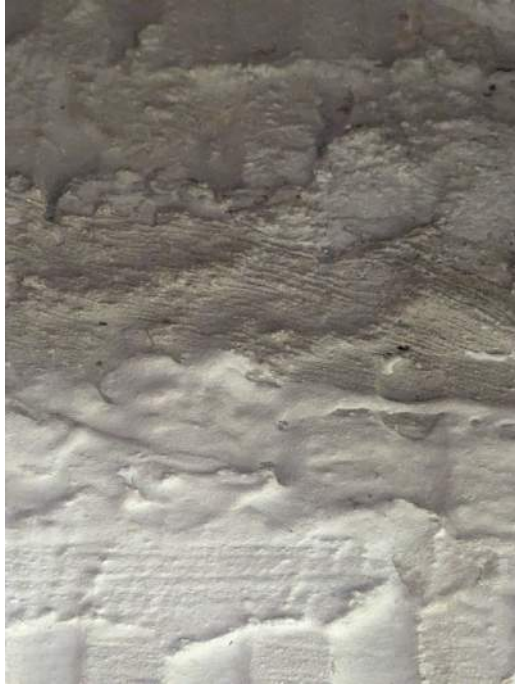
Photograph 21: HID 32. Interior Gray Coating (NAD) on Perimeter Walls
