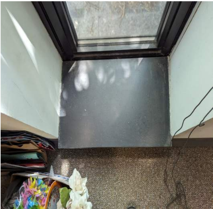
Photograph 15: HID 23. Black Cement Window Sill (ACM)
