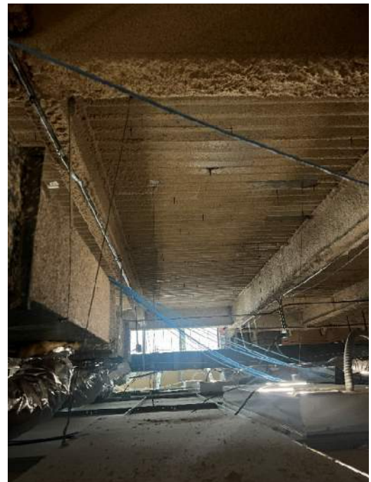
Photograph 32: HID 01. Tan Spray-Applied Fireproofing (NAD) View above drop ceiling.
