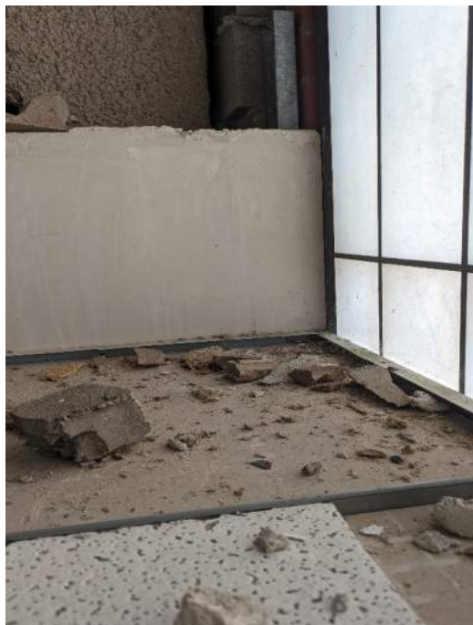
Photograph 9: HID 09. Brick (NAD) and Mortar (NAD)
