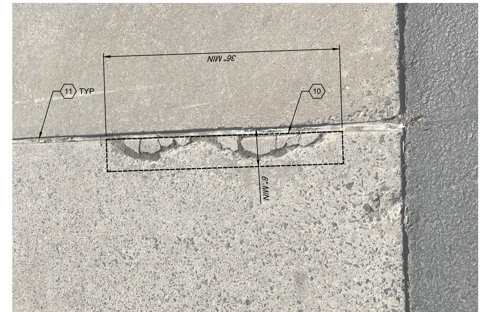
3 APRON REPAIR AREA #2 C-2 NOT TO SCALE
