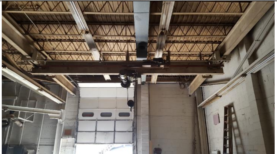
View of an electric winch located on the ceiling of the warehouse.
